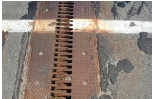
Non-Bicycle Compatible Bridge Expansion Joint
