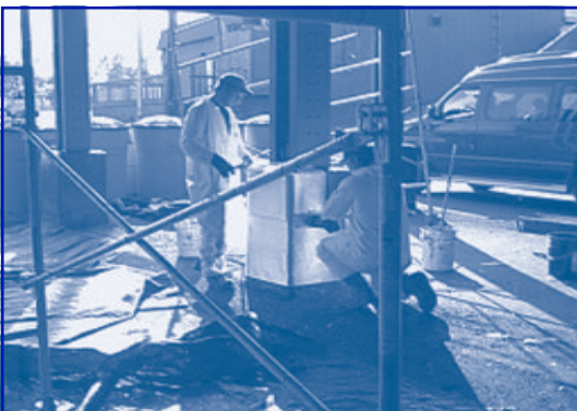
Concrete base wrapped with GFRP
