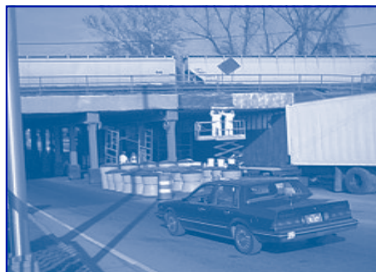
Finished left side with repair on right side
