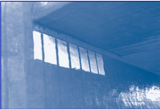
Abutment wall with primer
