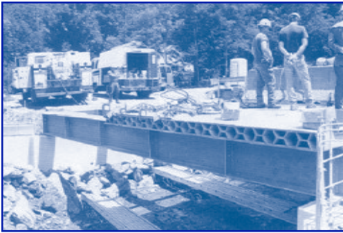
Wickwire Run Bridge during construction
