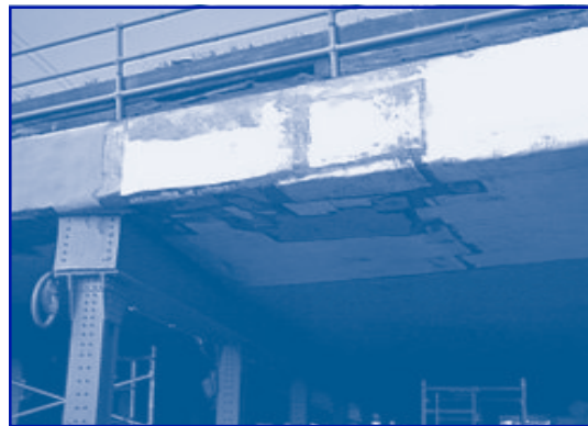
Viaduct roof with filler
