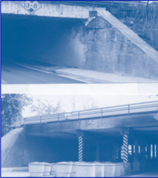
East Street Viaduct
