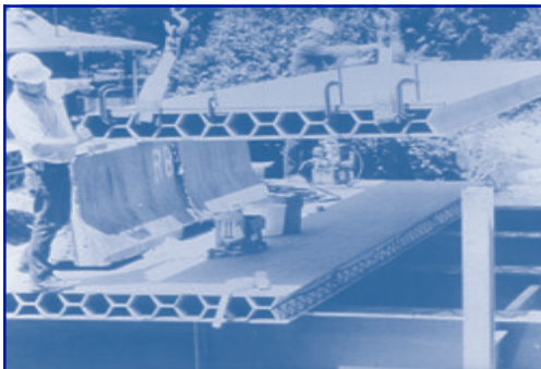
Placement of GFRP deck modules on steel girders
