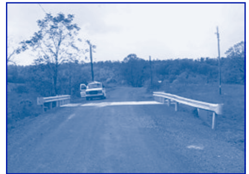
Driver's view of bridge
