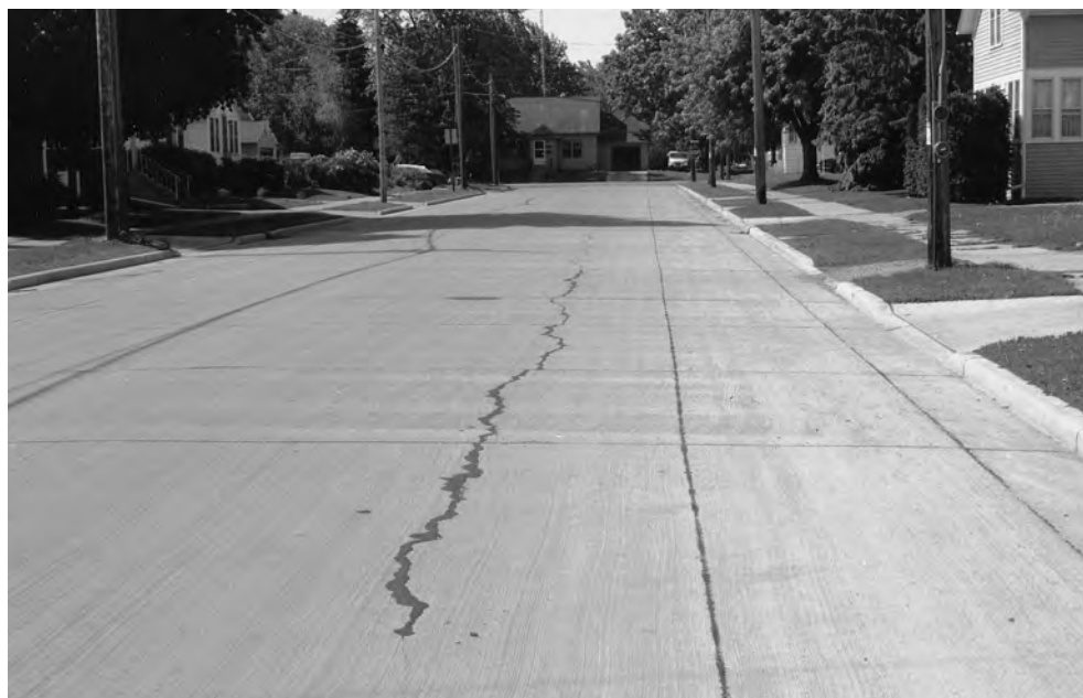
► Isolated meander crack, tight and well sealed.
