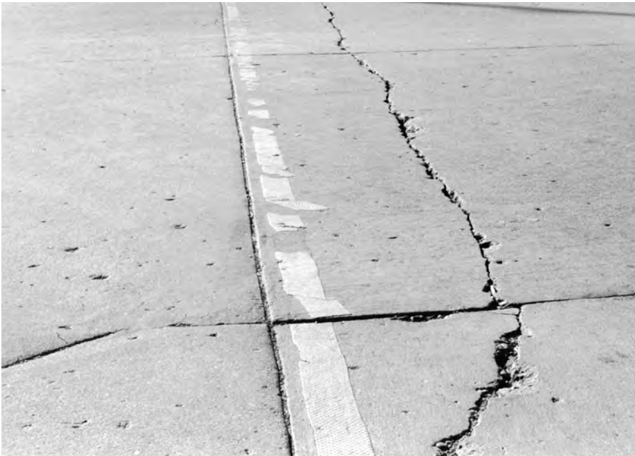
◀ Meander crack roughly parallel to longitudinal joint.
