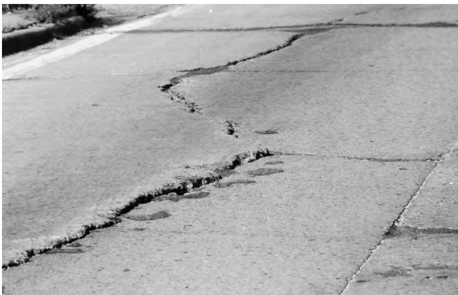
◀ Faulting and spalling of a meander crack.
