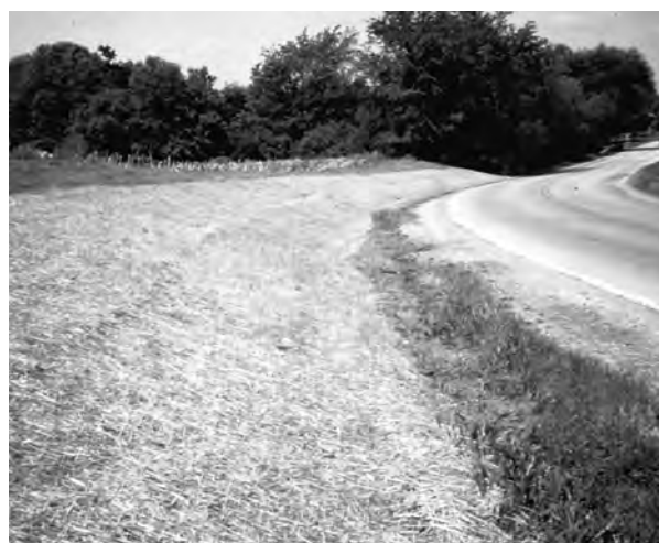
▲ Adequate rural ditch and good erosion control. RATING: Good
