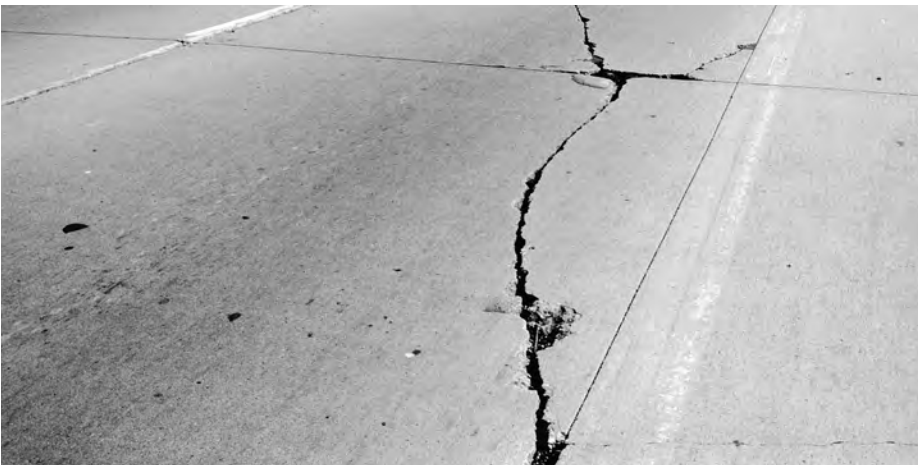
◀ Meander crack caused by settlement. Lack of maintenance allows water to intrude and debris to collect in crack.
