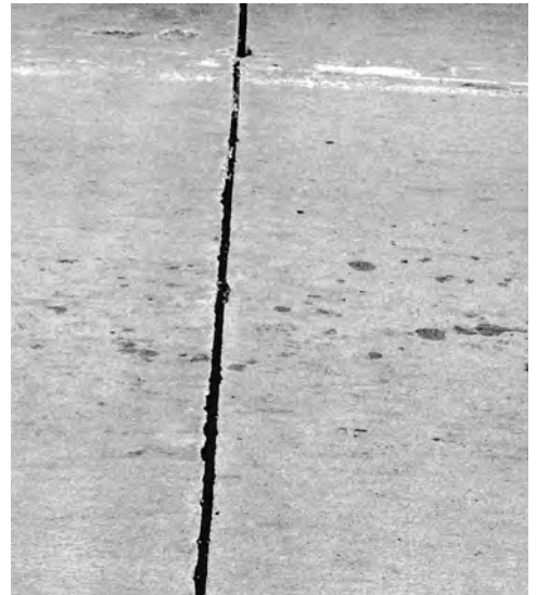
▲ Partial loss of joint sealant.
