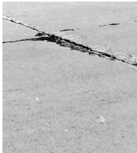
▼ Transverse joint has slight faulting and spalling.
