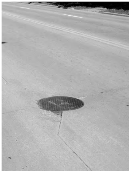
► Isolated spall at manhole.
