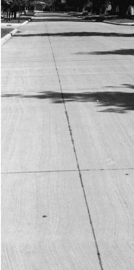
New, well-sealed longitudinal joint.
