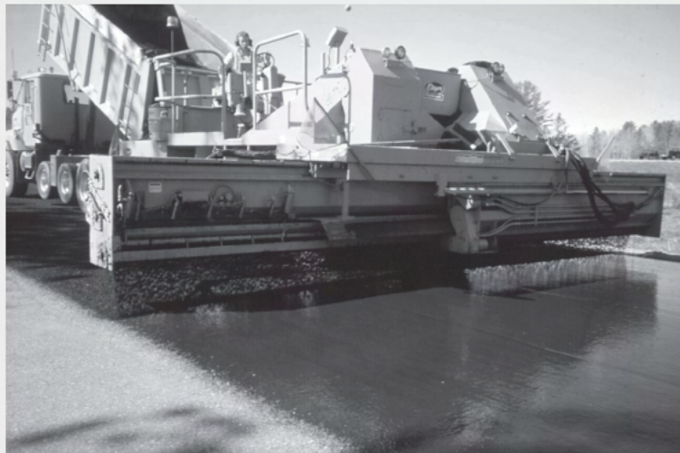
▲ Spreading cover aggregate
