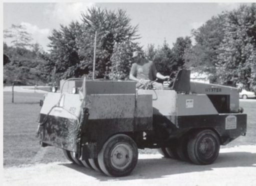
▲ Spreading cover aggregate
