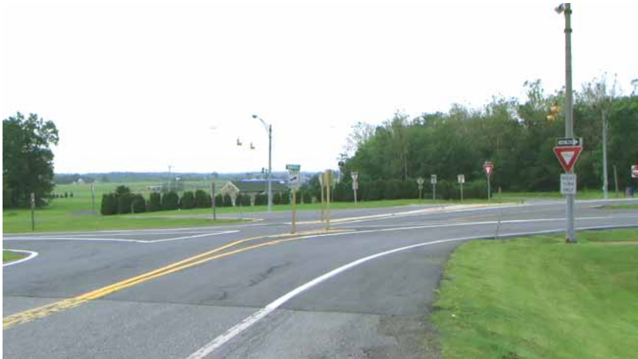
Figure 110. Photo. Signing and marking at an unsignalized J-turn in Emmitsburg, MD.
