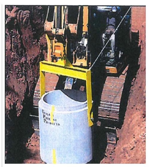
discovered that it was easier to transport, align, and level the manhole sections. Additionally, the lift took away the guess work of having to chain or worry about slippage while transporting and setting the unit.
