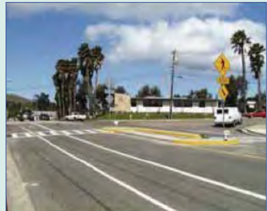
Z-Crossing, City of San Luis Obispo
