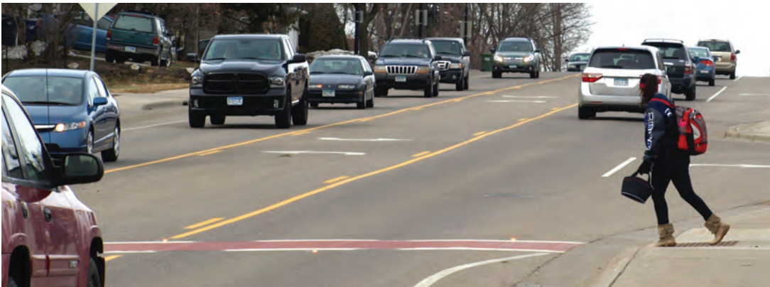
IN-ROAD WARNING LIGHTS
