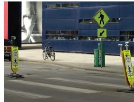
PEDESTRIAN CROSSING WARNING SIGN PLUS IN-ROAD SIGNS
