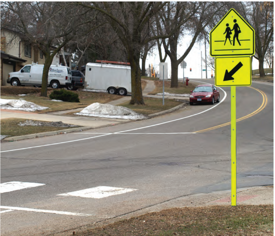
MARKED AND SIGNED SCHOOL CROSSING
