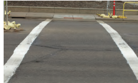
STANDARD/TRANSVERSE CROSSWALK PAVEMENT MARKINGS
