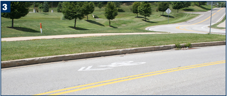
The gouges in the top of the curb indicate vehicles failing to negotiate the curve and running off the west side of the road.
