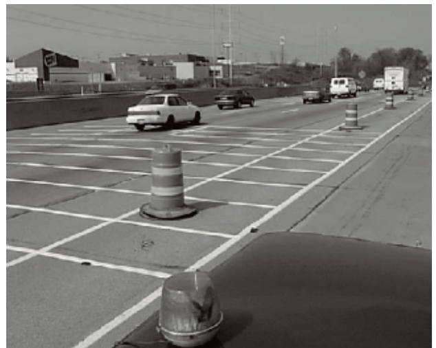
Rumble strip for work zone speed control
