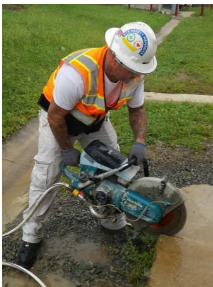
A construction worker using a handheld power saw with an integrated water delivery system.
