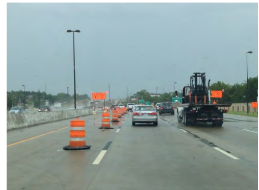
Figure 10. Oklahoma Work Zone in Wet Weather Conditions (Source: Leidos)
