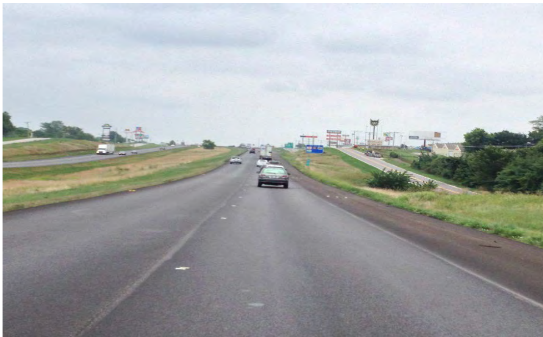
Figure 3. Use of Temporary Raised Pavement Markers on Centerline and Shoulder on I-70 in Missouri.
