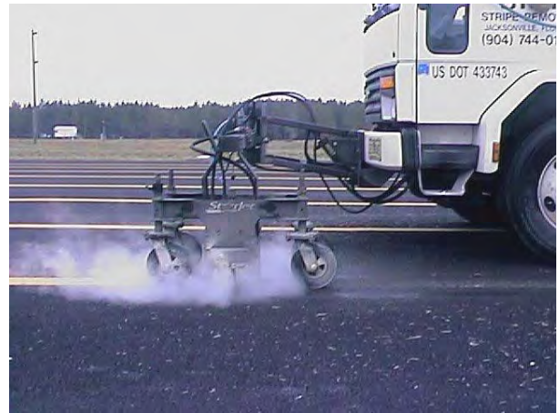
Figure 12. Example of Water-Blasting to Remove Striping in Florida (Source: FHWA, 2013)
