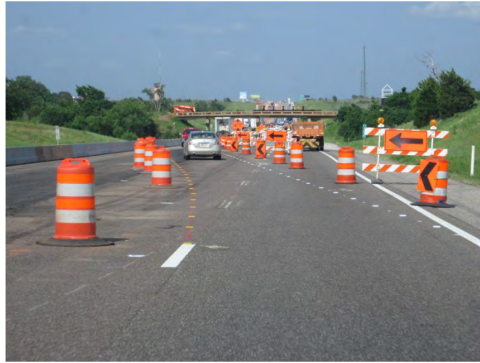
Figure 4. Use of Temporary Raised Pavement Markers on Lane Shift on I-44 in Oklahoma. (Source: Leidos)
