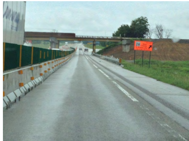
Figure 9. Use of Tabs on Barrier and Paint Wear on Edge Line on I-44 in Oklahoma
