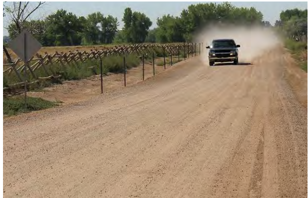
Figure 41. Photo. Dusty when dry.
