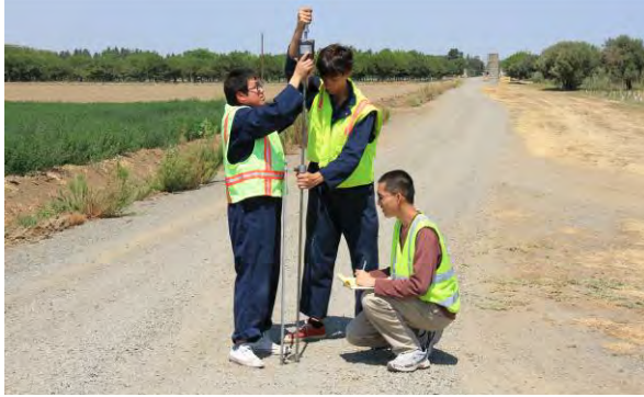
Figure 86. Photo. Checking layer depths with dynamic cone penetrometer.
