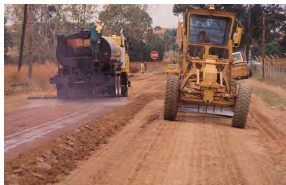
Figure 14. Photo. Mix-in treatment.
