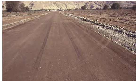
Figure 52. Photo. Electrochemical additive.
