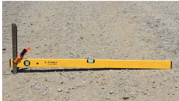
Figure 89. Photo. Checking crown with a simple level.
