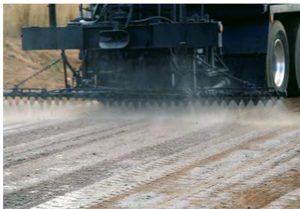
Figure 72. Photo. Penetration with pre-wetting.
