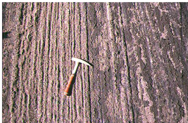
Figure 71. Photo. Poor penetration without pre-wetting.
