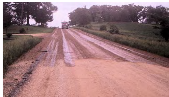
Figure 29. Photo. Lignosulfonate road.
