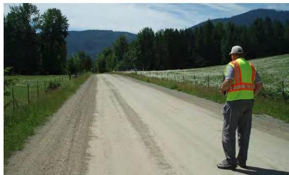
Figure 25. Photo. Keeping a good road good.
