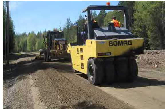
Figure 80. Photo. Compaction with rubber-tired roller.
