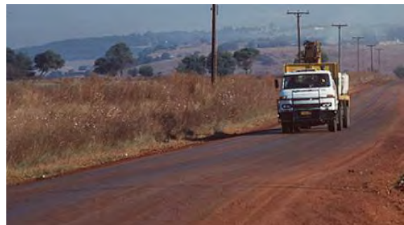
Figure 91. Photo. Road after treatment.
