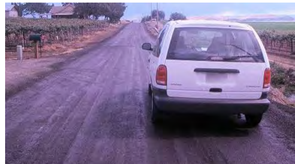
Figure 81. Photo. Completed road.
