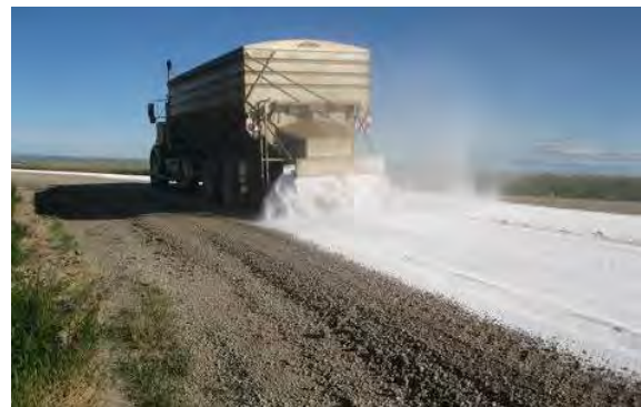
Figure 75. Photo. Flake application of calcium chloride.
