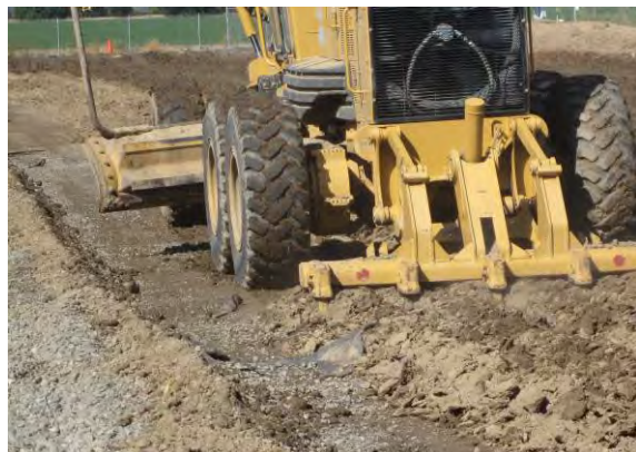
Figure 78. Photo. Ripping with a grader.
