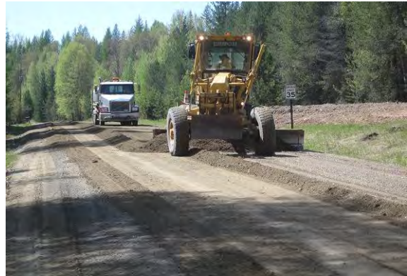
Figure 16. Photo. Maintenance of treated road.
