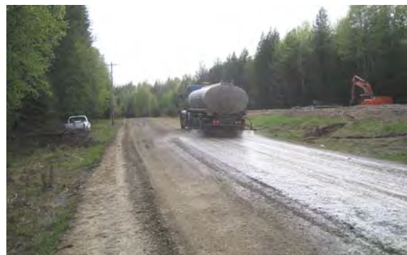
Figure 13. Photo. Spray-on treatment to well-prepared road.
