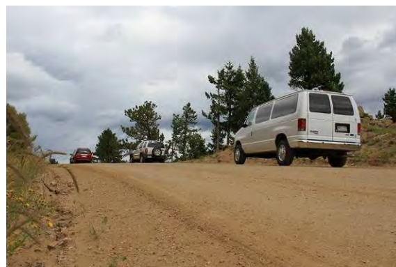
Figure 60. Photo. Good crown (4 to 6%).
