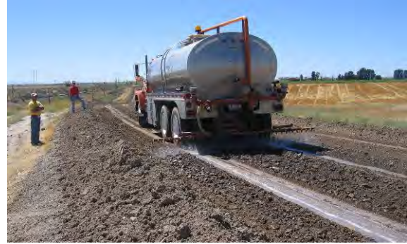
Figure 79. Photo. Spraying the additive.
