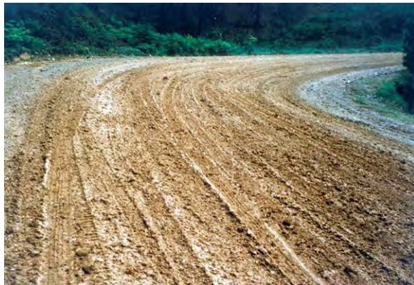
Figure 42. Photo. Slippery when wet.
