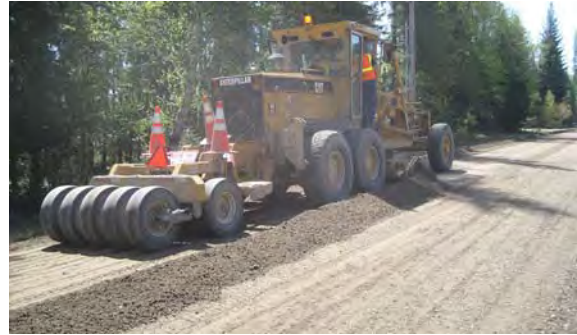
Figure 9. Photo. Grader maintenance.
