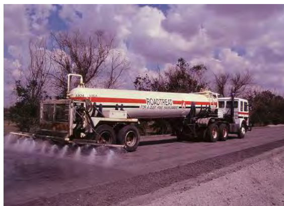
Figure 97. Photo. Road preparation to minimize environmental impact.
