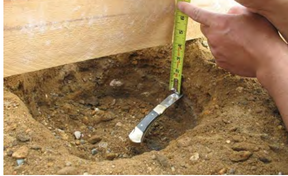
Figure 87. Photo. Checking gravel thickness.
