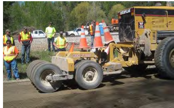
Figure 65. Photo. Grader-mounted roller.
