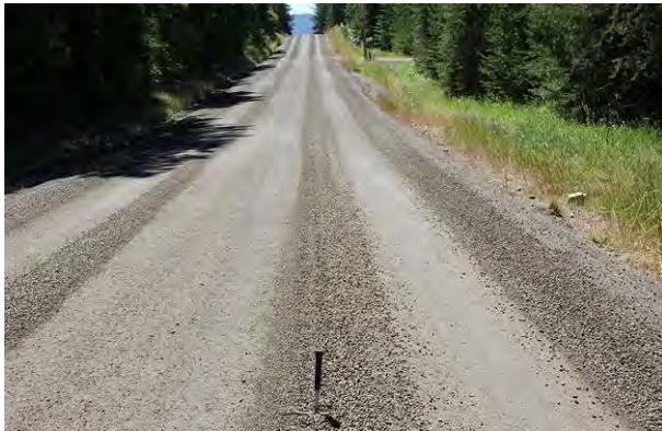
Figure 40. Photo. Raveling.
