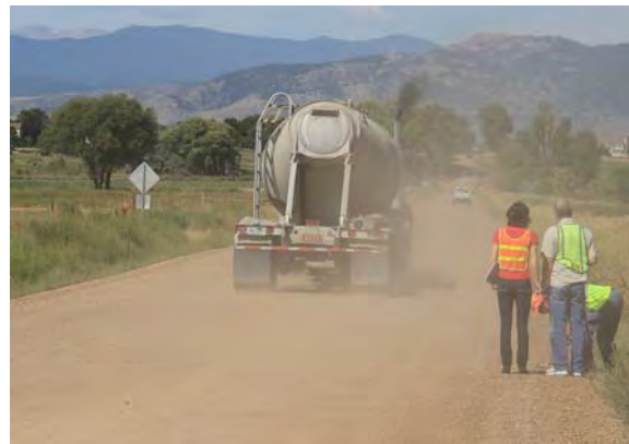
Figure 24. Photo. Acceptable dust level.
