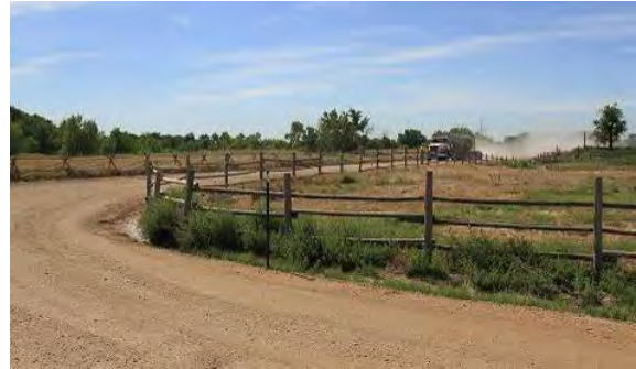
Figure 68. Photo. Very sharp curve.
