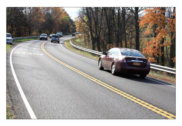
Center line rumble strips are placed as a countermeasure for driver error, rather than roadway deficiencies. They are designed primarily to assist distracted, drowsy or otherwise inattentive drivers who unintentionally stray over the center line. For this set of drivers, the
