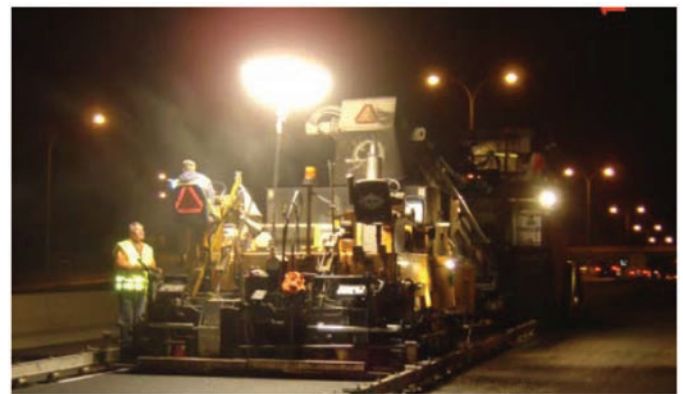
Figure 4 - Balloon Lighting in a Nighttime Work Zone
