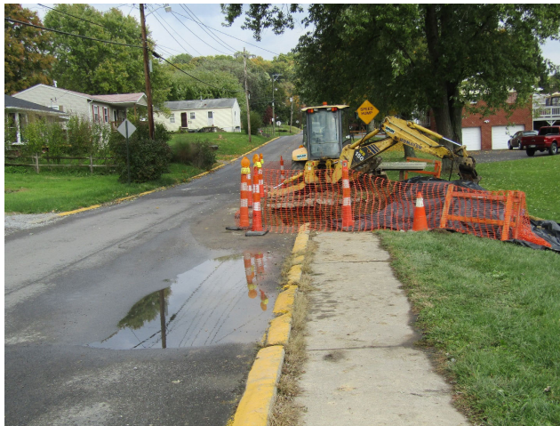
Approaching the Work Area
