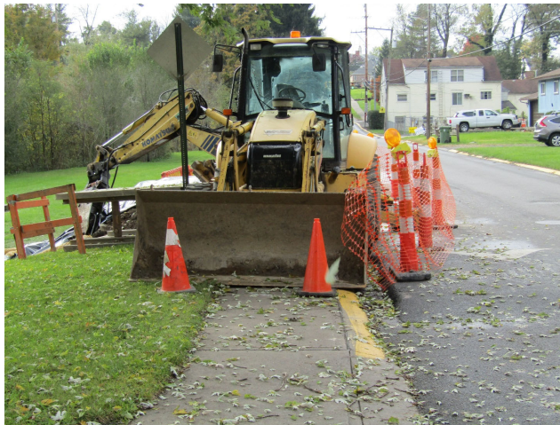
Close-Up View Looking West
