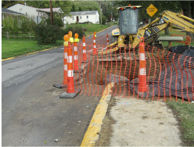
Close-Up of Work Area
