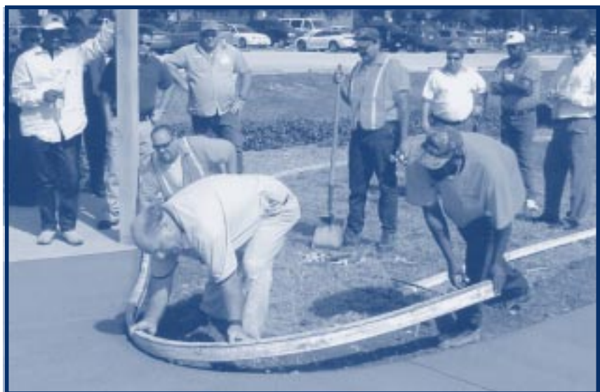
Gary Vroman and Crew removing the form boards.
