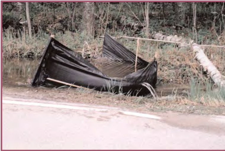
Silt fence as temporary ditch check.
