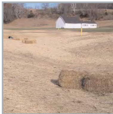
Hay bales were used in the ditches to reduce flow velocity.
