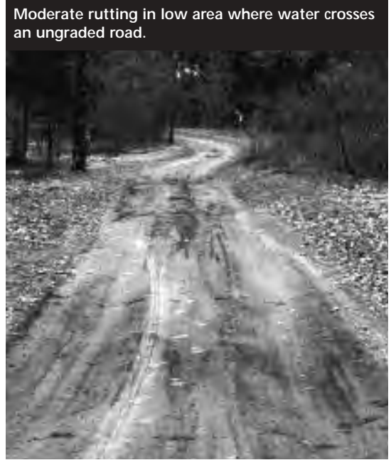
Severe rutting makes travel difficult.
