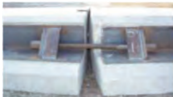
Figure 4. Section Connecting Pin (Florida Design)
