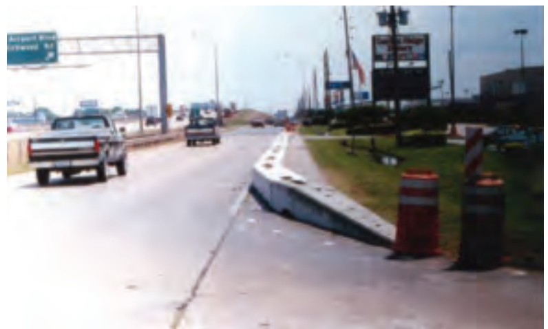
Figure 3. LPB with End Terminal
