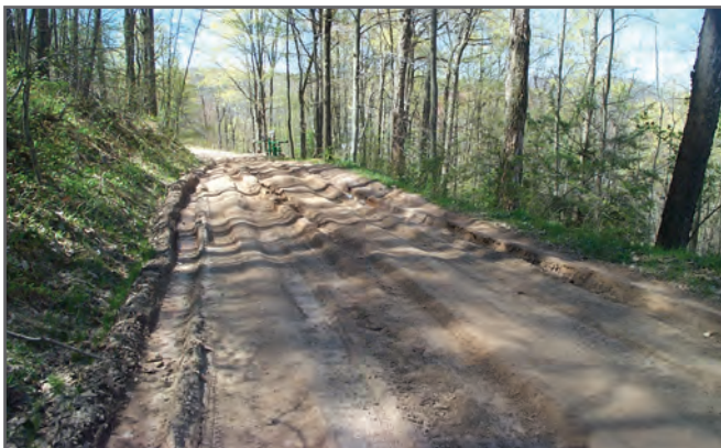
Figure 2—This road had rutting in the surface due to a lack of surface aggregate, excessive clay, poor compaction, and poor road surface drainage combined with weak subgrade soils.
