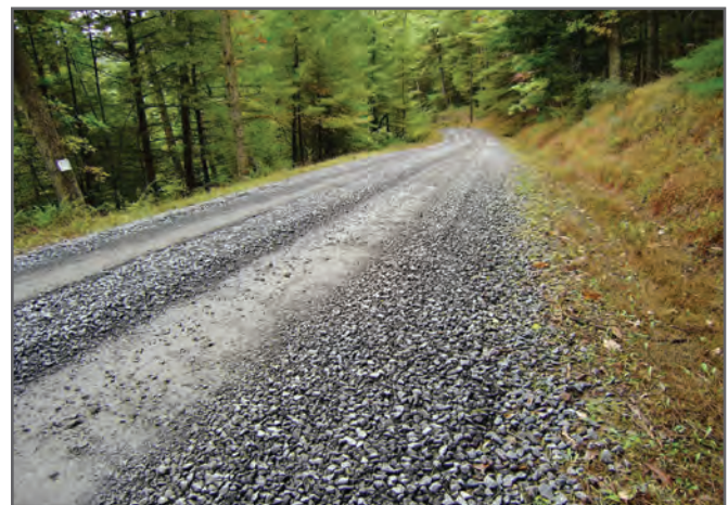
Figure 3—Lack of road surface drainage in conjunction with a poor aggregate gradation can create potholes that can weaken the structural section of the road. Ensure that any ruts and potholes are reprocessed and compacted before placing any new aggregate.
