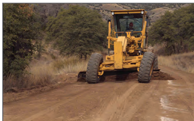
Figure 8—The grader operator is sometimes blamed for gravel maintenance/rehabilitation problems when the actual problem is often material related.
