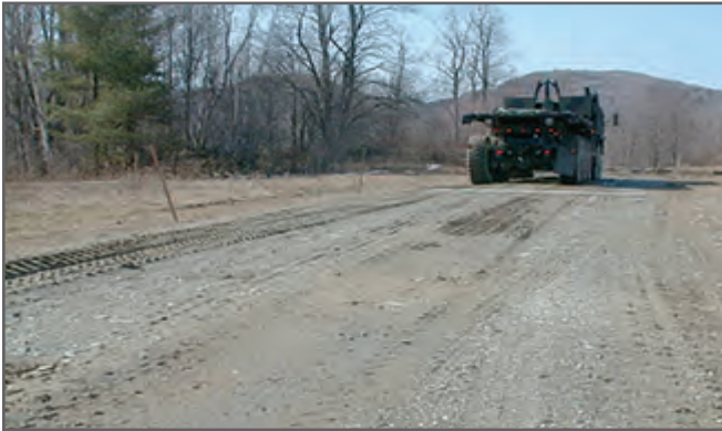
Figure 3—Lack of road surface drainage in conjunction with a poor aggregate gradation can create potholes that can weaken the structural section of the road. Ensure that any ruts and potholes are reprocessed and compacted before placing any new aggregate.
