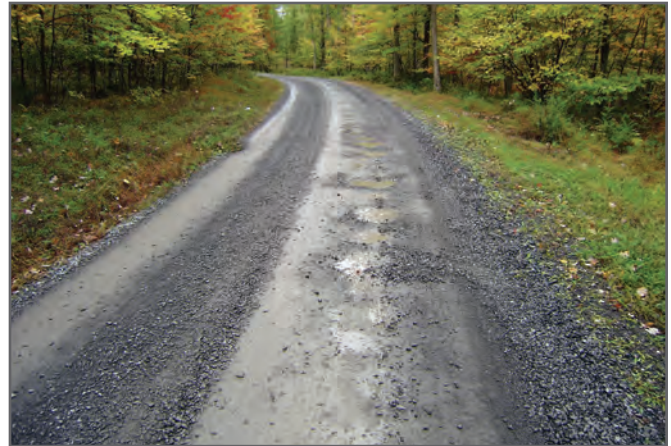
Figure 3—Lack of road surface drainage in conjunction with a poor aggregate gradation can create potholes that can weaken the structural section of the road. Ensure that any ruts and potholes are reprocessed and compacted before placing any new aggregate.
