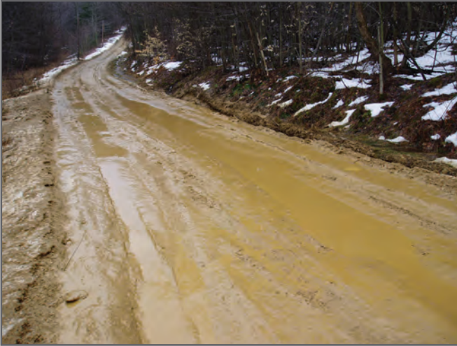
Figure 5—Too much clay or the use of low-durability aggregate in the surface aggregate can lead to the retention of excessive moisture and can cause rutting, excessive runoff, surface deformation, and damage to the road, especially during thaw cycles and after rain events. Good roadway surface and subsurface drainage are the most cost-effective actions to take to maintain or improve the quality and strength of any soil or aggregate.
