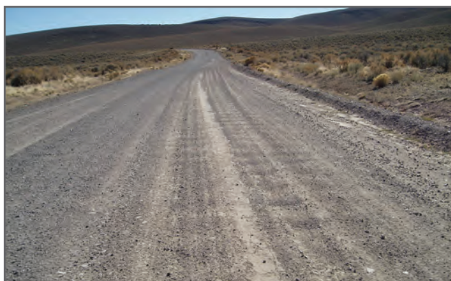
Figure 7—This road had corrugations (washboarding), which resulted from insufficient fines in the surface aggregate (as well as lightweight traffic and lack of timely maintenance). Corrugations and washboarding can be removed temporarily by grading. However, the real problem is an insufficient amount of fines and/or no plasticity.
