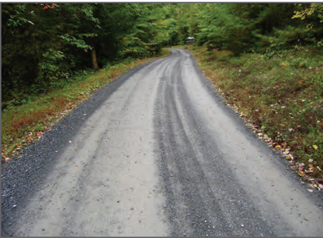
Figure 10—These roads had well-compacted surfacing materials with an appropriate gradation of aggregates and a sufficient amount of fine material.
