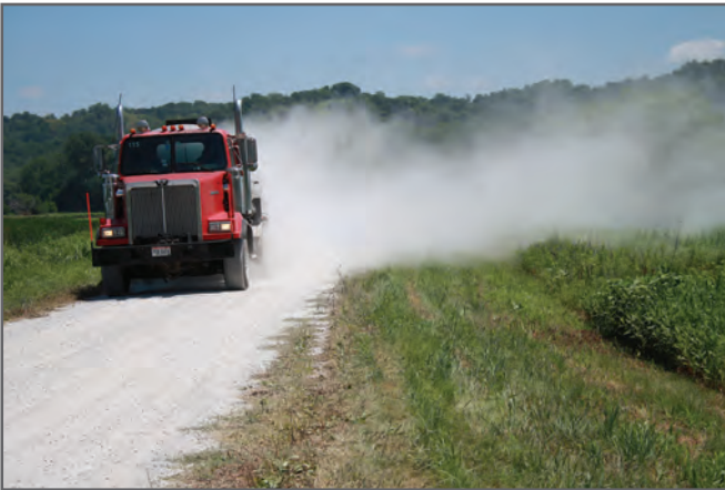
Figure 6—Too much clay within the surface aggregate can migrate to the surface of the aggregate, thereby increasing the amount of sediment runoff during rain events and the amount of dust during dry conditions.
