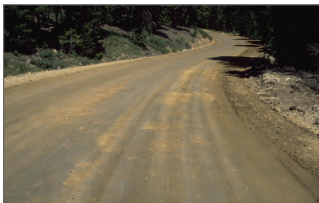
Figure 9—The use of high-quality aggregate surfacing will resist erosion, make it reasonably firm, perform well, and stretch the life cycle before regraveling is needed. A well-maintained road, particularly with a dust palliative, reduces road user costs, prevents road damage, and minimizes sediment production.
