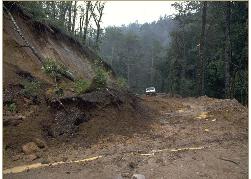
This photo by Gordon Keller shows a slope failure, a common problem.
