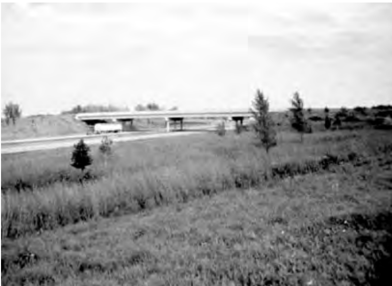
Prairie Restoration Project on Interstate 90
