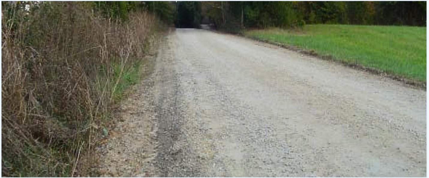
Photo by the FHWA "Gravel Roads Construction & Maintenance Guide"
