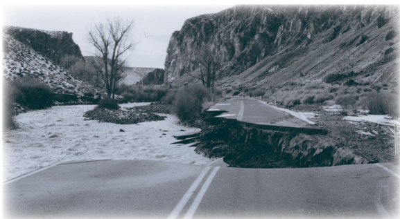
Figure 1. The results of a culvert failure.
