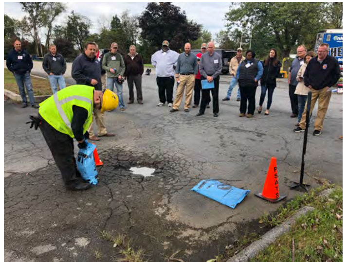
Cold mix patching materials were some of the products demonstrated.
