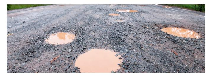
can return lost stone from the shoulders and reshape the cross section at significantly less cost.
