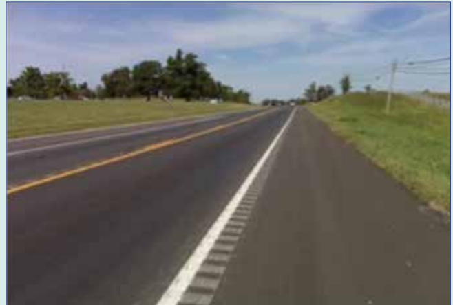
Figure 2. Shoulder rumble stripe
