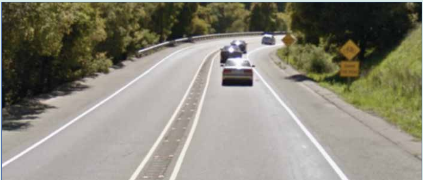
Figure 3. SR 84, courtesy of Google street view
