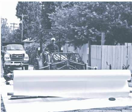
As shown in this photo, the mat comes on a large roll and is rolled out using a special attachment on a standard tractor.
