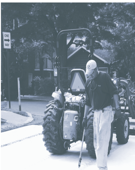
The TruPave® mat is laid before the asphalt is applied. The mat acts as a moisture barrier and helps to reduce reflective cracking.
