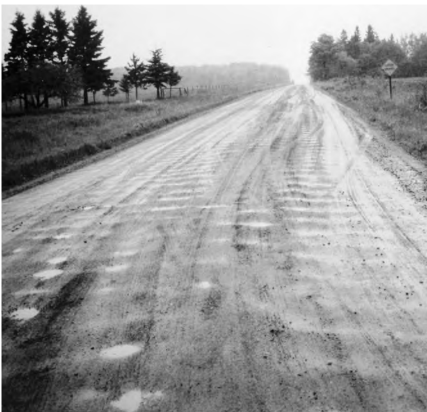
► Severe washboarding traps water.
