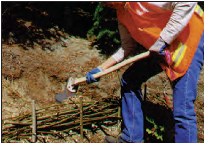
Figure 15—Brushlayer modified with willow fencing. (Lewis 2000)
