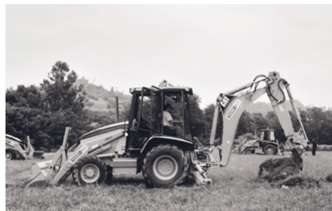
Richard Vandevender, from the City of Elkins, begins digging his trench.
