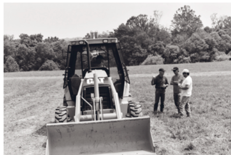
Dee Hadfield explains a backfilling and leveling technique.
