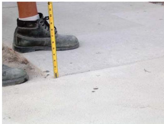
*The top photo illustrates a 1 inch trip hazard in a sidewalk. The bottom photo shows the results after using GrindAll.*
